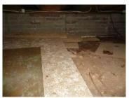
Water pooling in the subfloor along the foundation wall can create a damp area conducive to termites.
