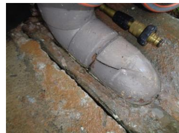
Downpipe cracked
