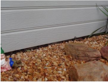
Garden covering foundation wall
