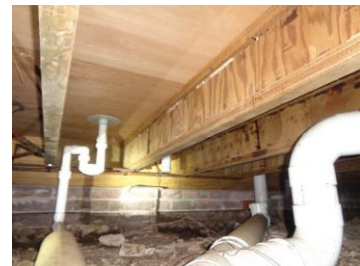
No leaking from wet area
