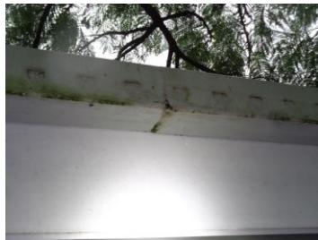
Gutter leaking
